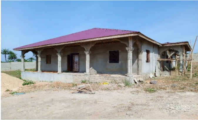
Unfinished Gbogbafeh Women's Multi-purpose Complex in Njagbwema.
