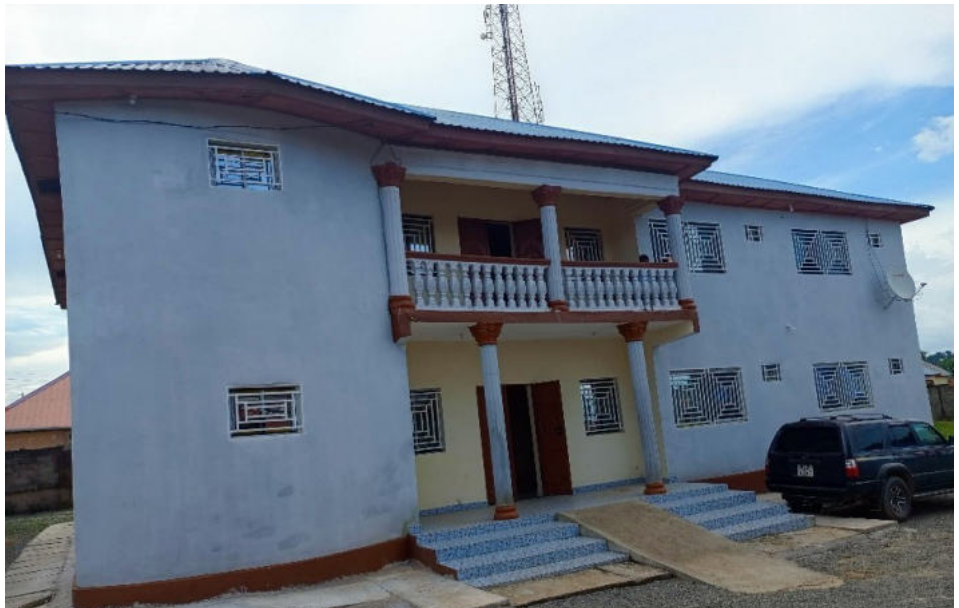
Tankoro CDC Secretariat and office of the Paramount Chief of Tankoro Chiefdom. Constructed by the CDC with funds from Koidu Limited mining company.
