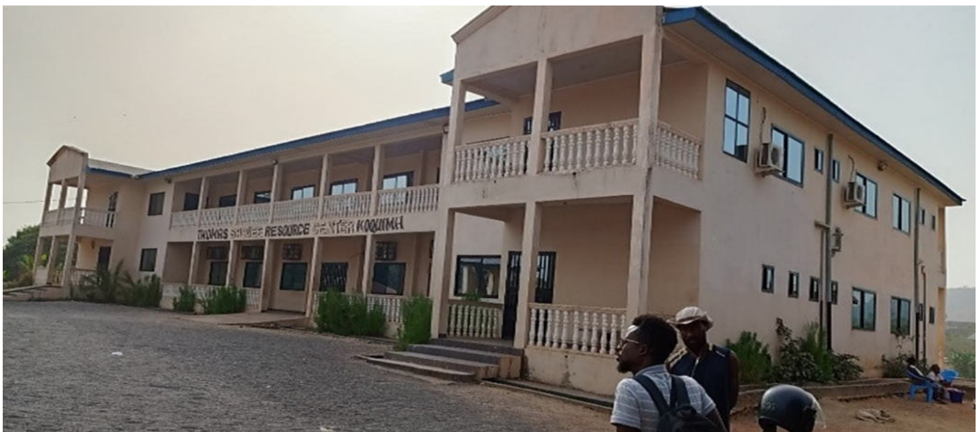
Thomas Saquee Hall constructed by Tankoro CDC.
